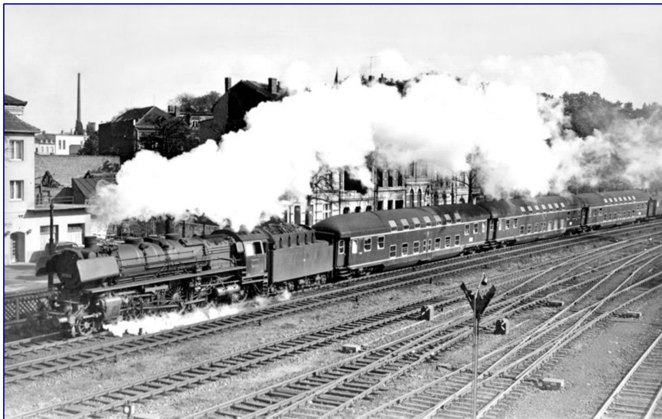
At the level of the Bonn freight station 03 1014 (Bw Dortmund Bbf) steams past on 4 October 1952 with E 719 (Frankfurt - Dortmund). The newly developed double-decker coaches are located in the train with retracted end entries at the end of the coach and a middle entry in the lower area. Photo: Carl Bellingrodt, Eisenbahnstiftung
